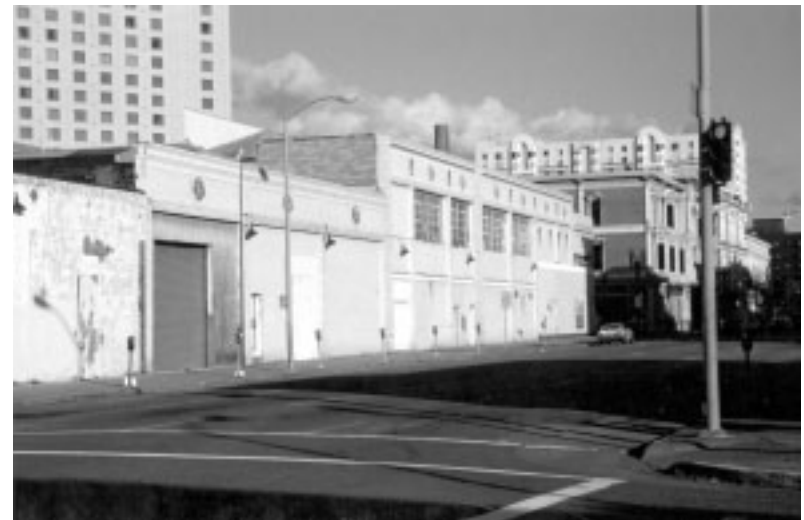
Rear facades with no street activity prior to re-use
